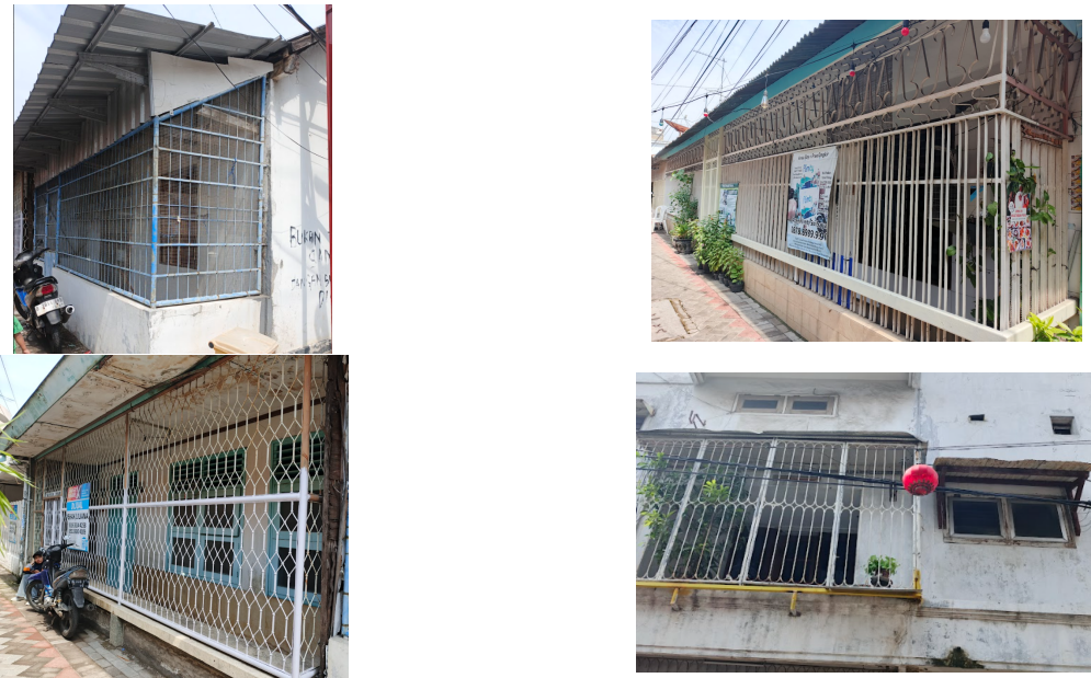
Figure 1. Fence with semi-permeable materials, such as iron bars or latticework in Kapasan Chinese Settlement
