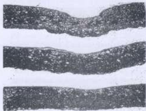
Figure 1. Cross section of hot mix macadam 14 mm asphalt pavement reinforced with geosynthetic grid following trafficking. Top Figure - without grid, Middle Figure - grid at mid depth of asphalt layer, Bottom Figure - grid at underside of asphalt layer.
